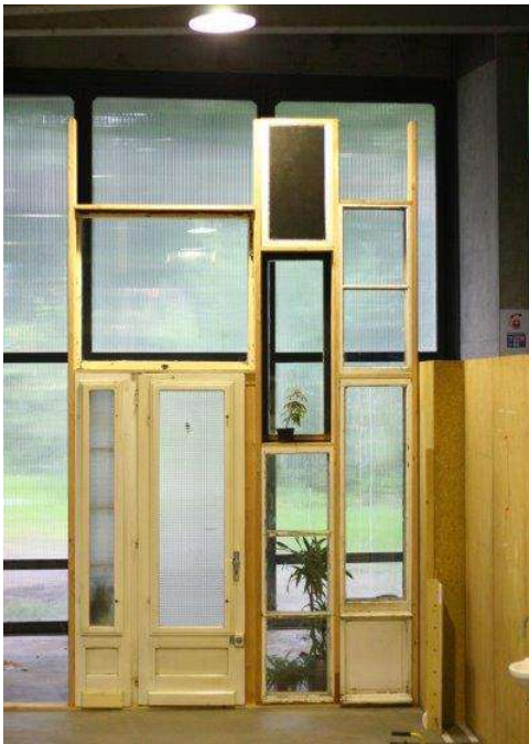
Scale 1/1 prototype reusing existing windows
